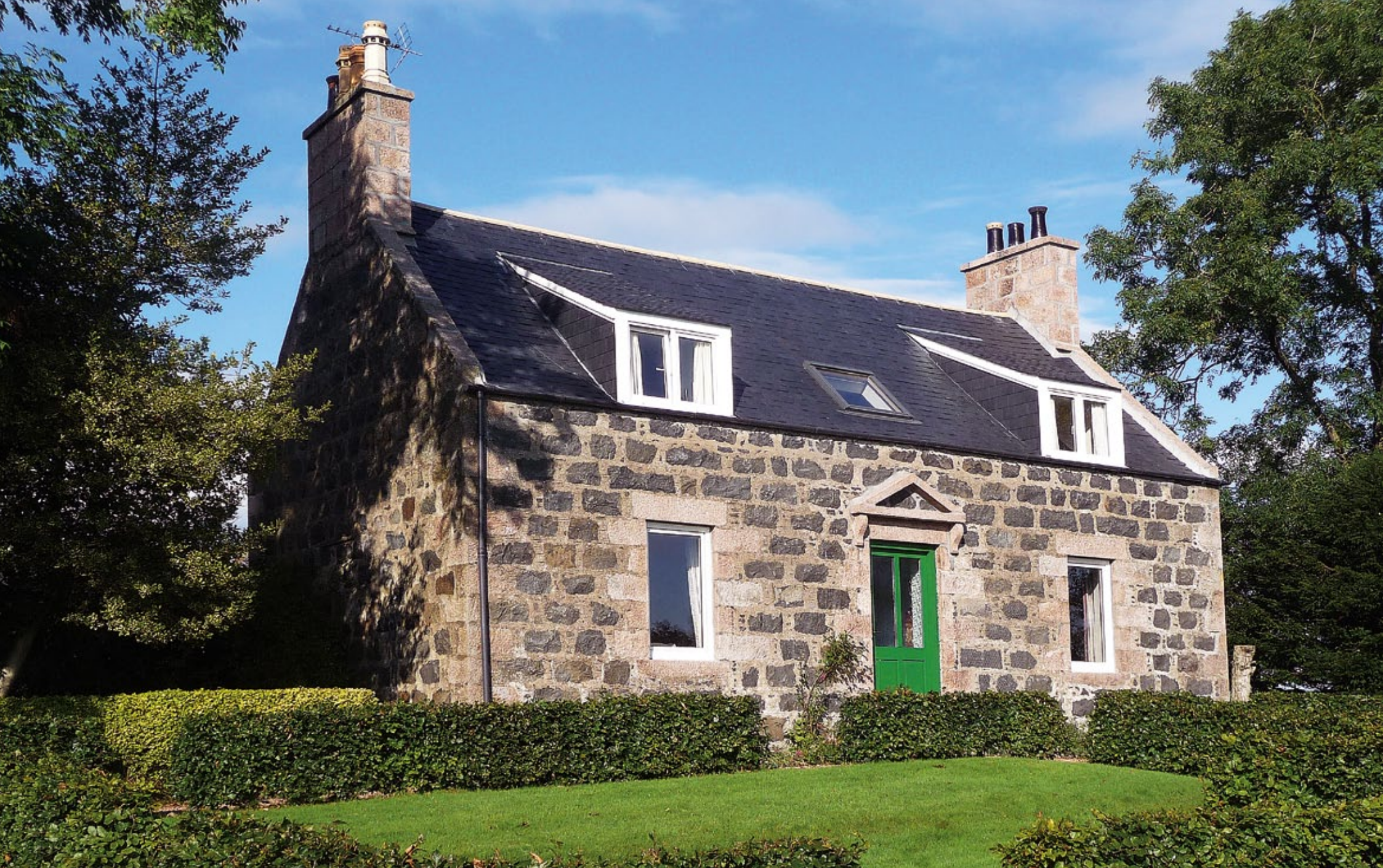
Knockolochie Farmhouse , Pitcaple, Aberdeenshire
