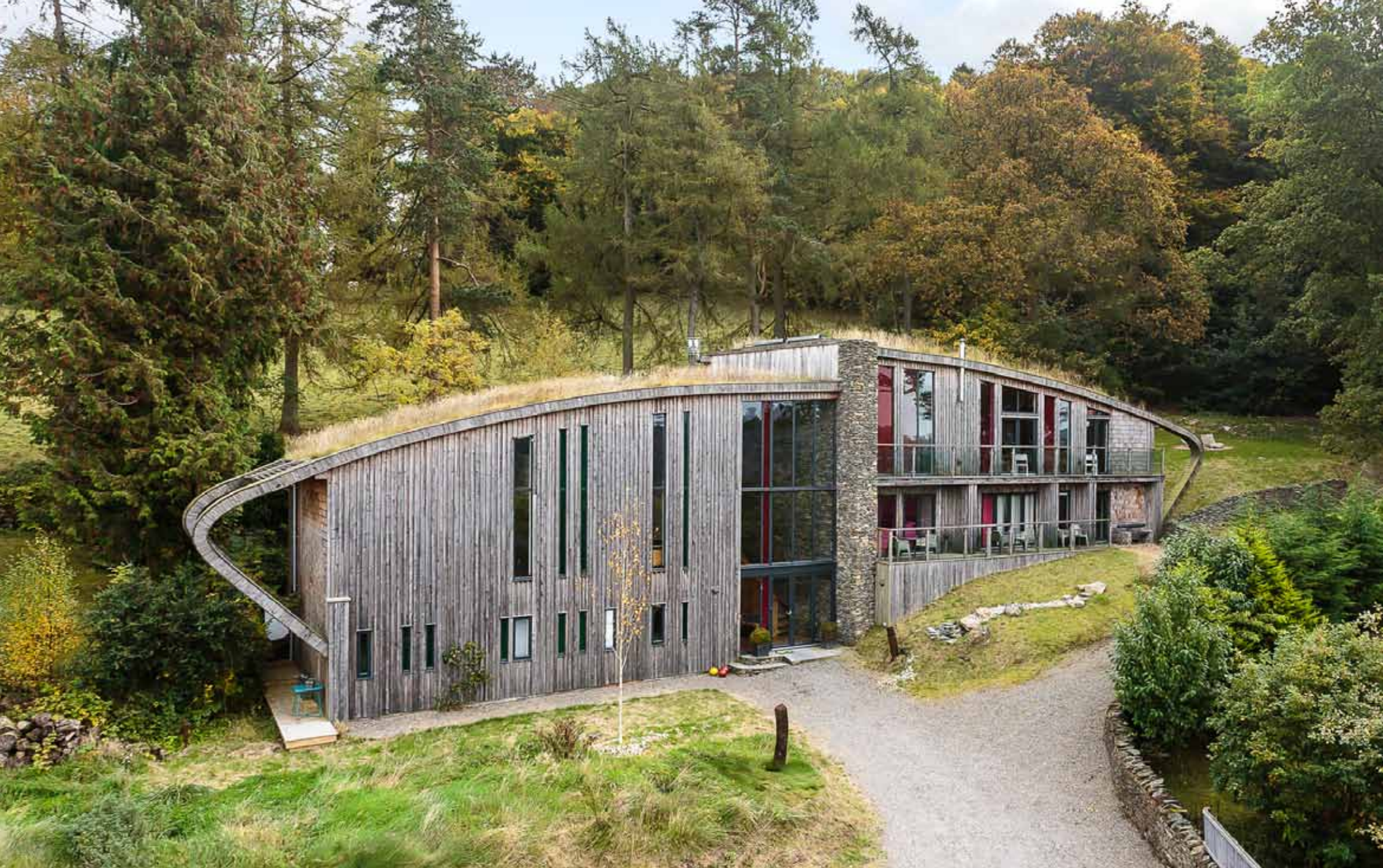
Dome House Brantfell Road, Bowness-on-Windermere, Cumbria
